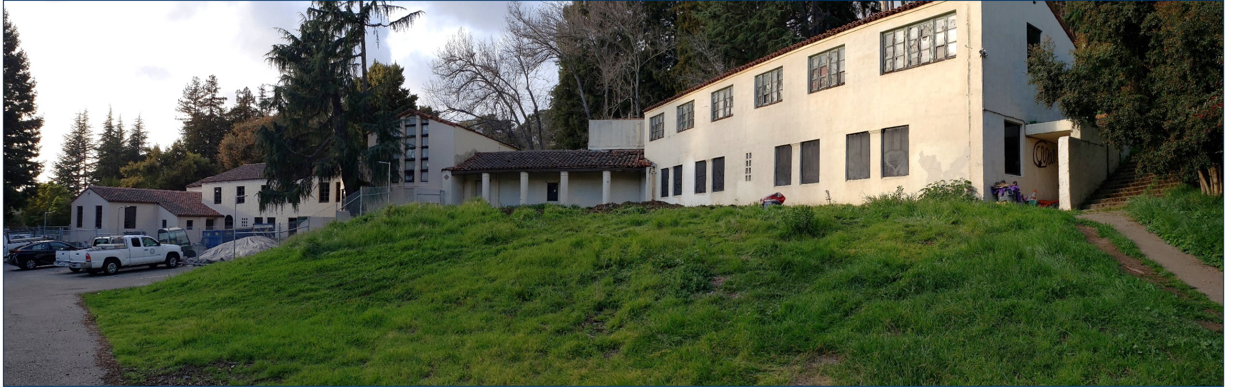
Image: Building 21, existing conditions, northwest wing removed (2019)
