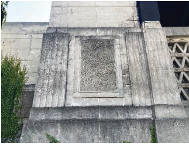
Concrete ornamentation base, panel, and fluted pilaster detailing
