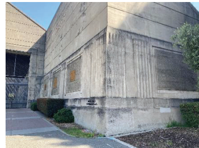
Concrete base detailing continued at south end of west bleachers
