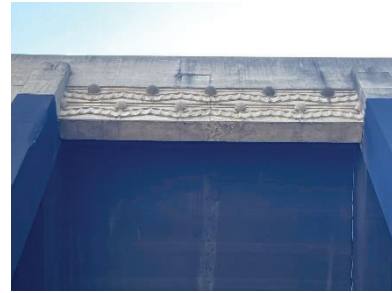
Concrete ornamentation detailing along top of west bleachers structure
