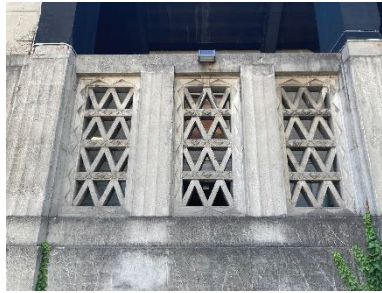
Concrete ornamentation screens along west bleachers
