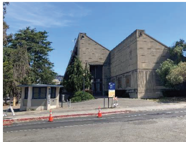
Angular massing of south end of west bleachers
