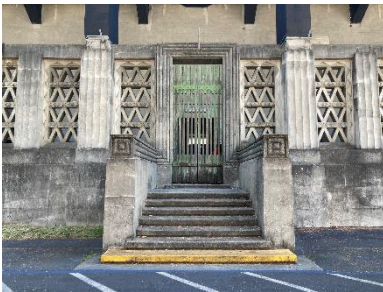
Concrete stairs and concourse gates
