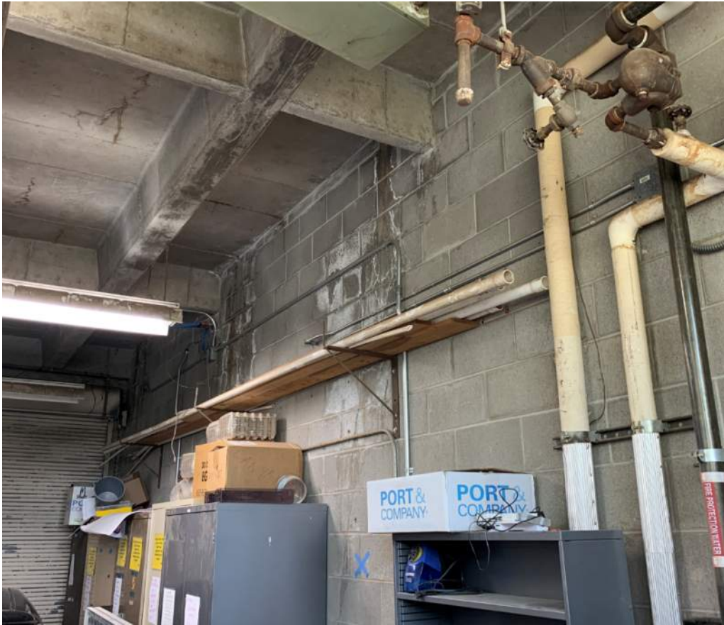
Figure 4 Non-load bearing CMU partition wall at the second story
