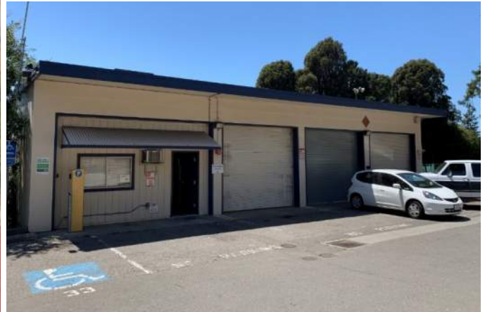
East Elevation Photo
