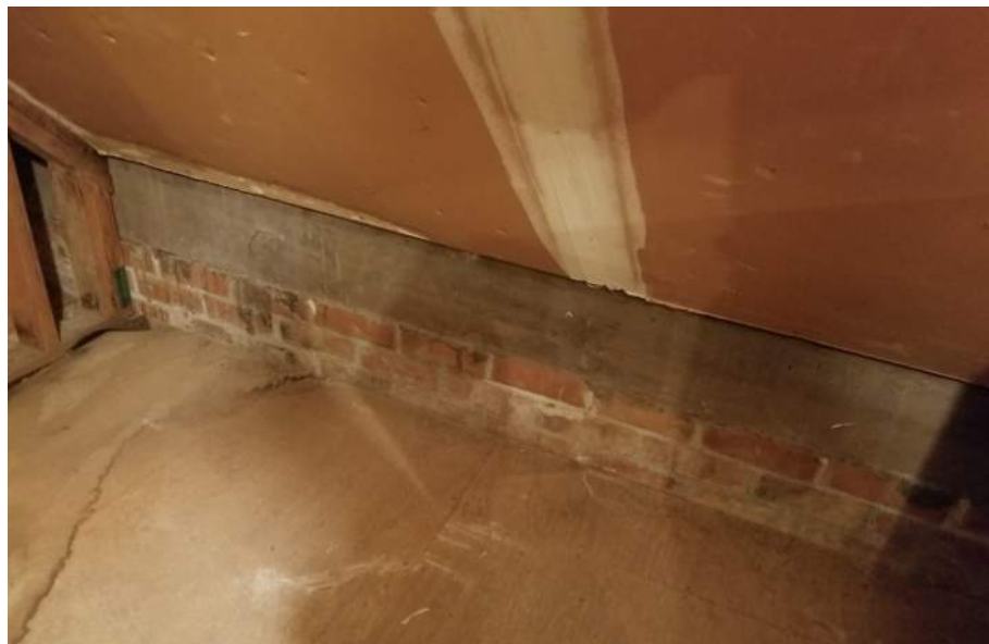
Concrete bond beam at top of masonry wall at Attic Level
