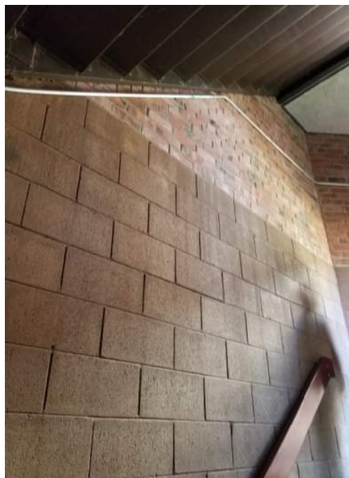
A combination of coneret masonry at the Basement and brick masonry at the upper levels ahs been used in Karpe Hall
