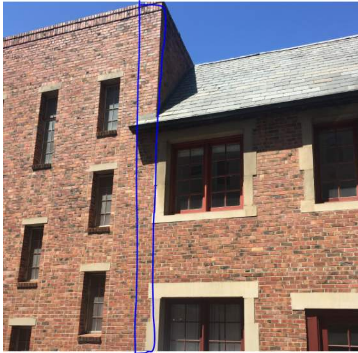
Shared masonry wall between Johnston Hall and Library Stacks
