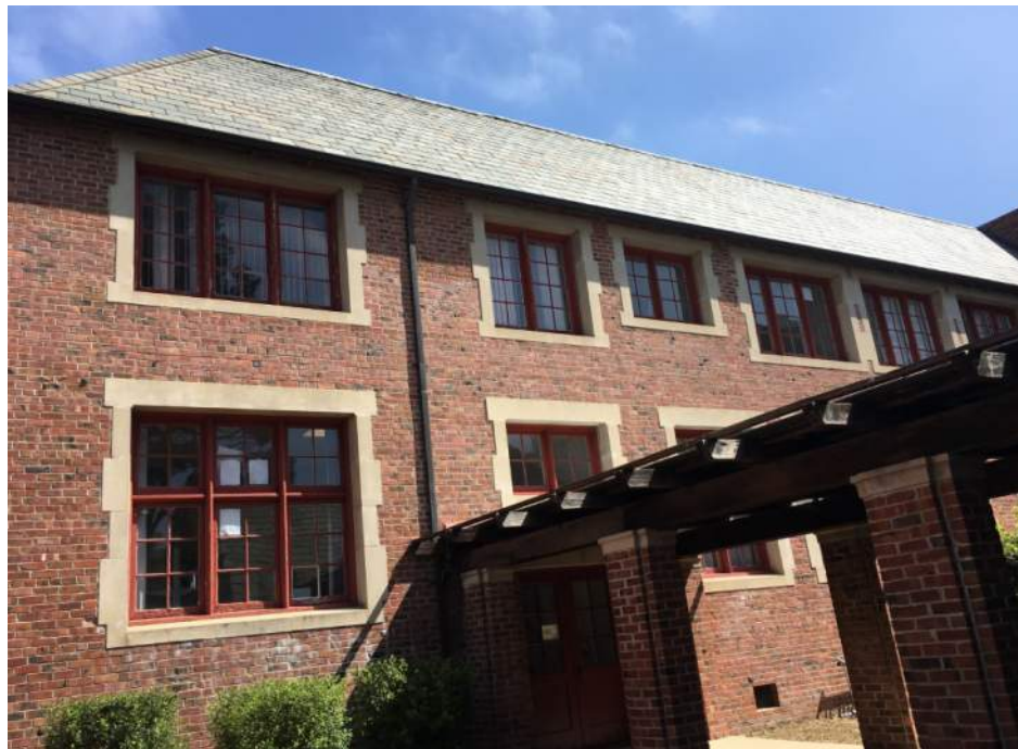
South side exterior wall with window openings
