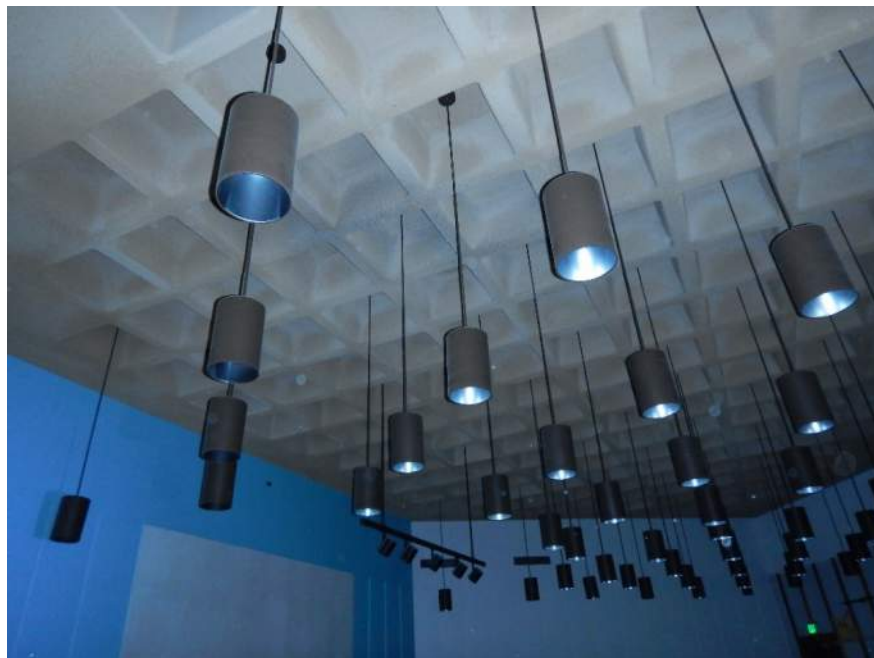
Figure A.3 Typical waffle slab
