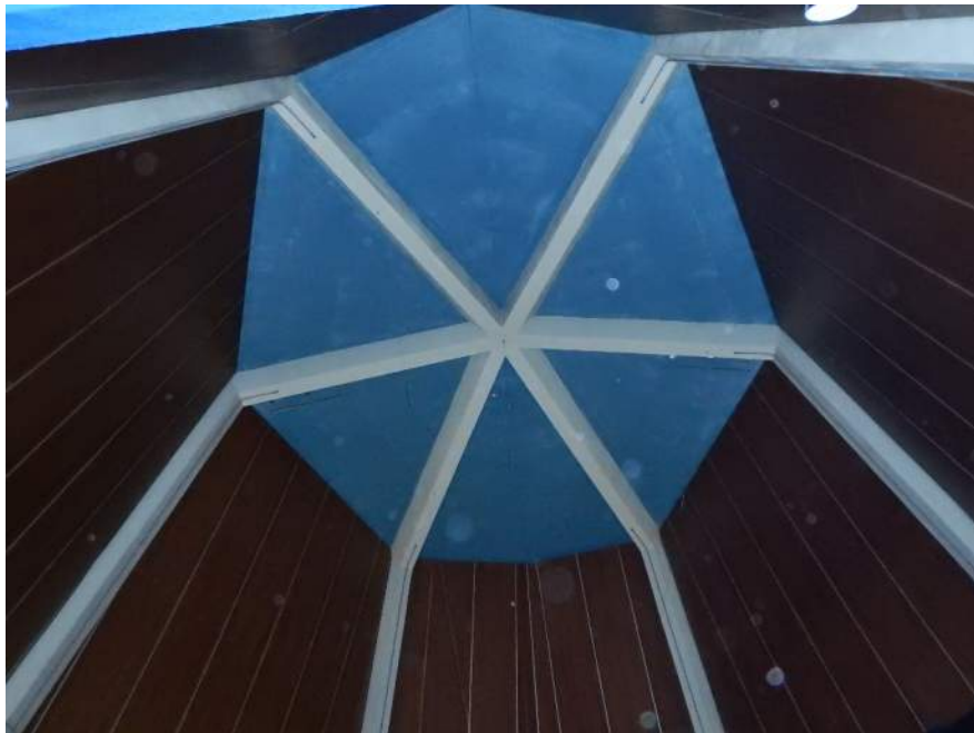
Figure A.2 Roof of Memorial Room in Information Center
