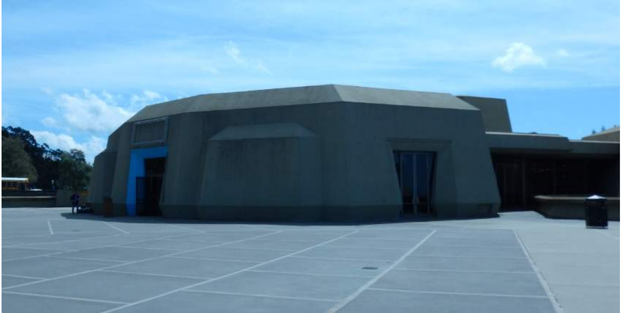
Figure A.1 Entrance Foyer at Level A at building exterior
