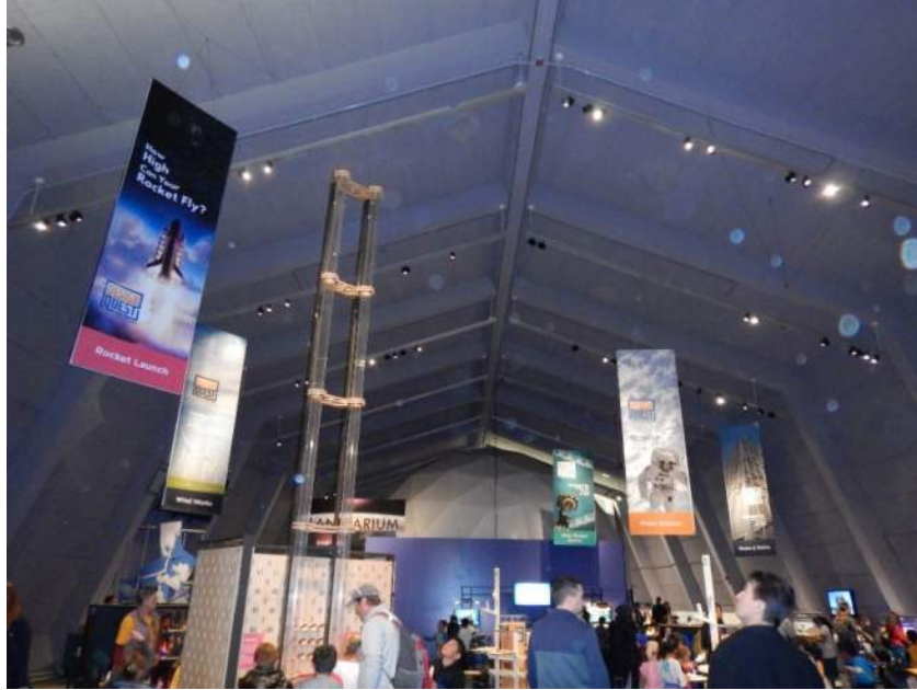
Figure A.1 Roof of Exhibition Hall
