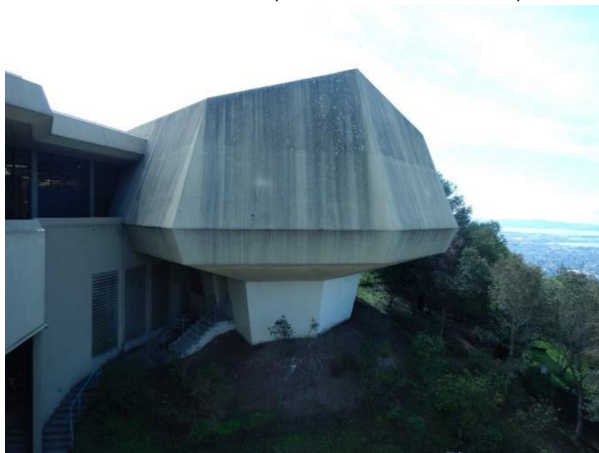
North Elevation Photo (Inverted Pendulum Structure)
