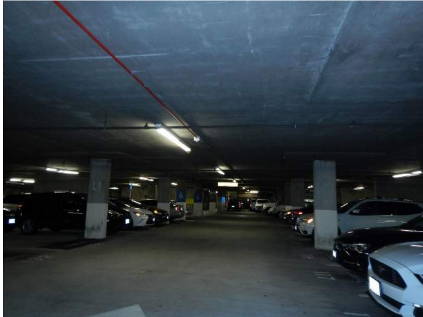
Figure A.3 Flat slab at parking levels
