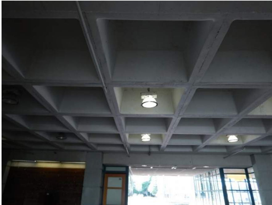
Figure A.1 Typical waffle slab at floors
