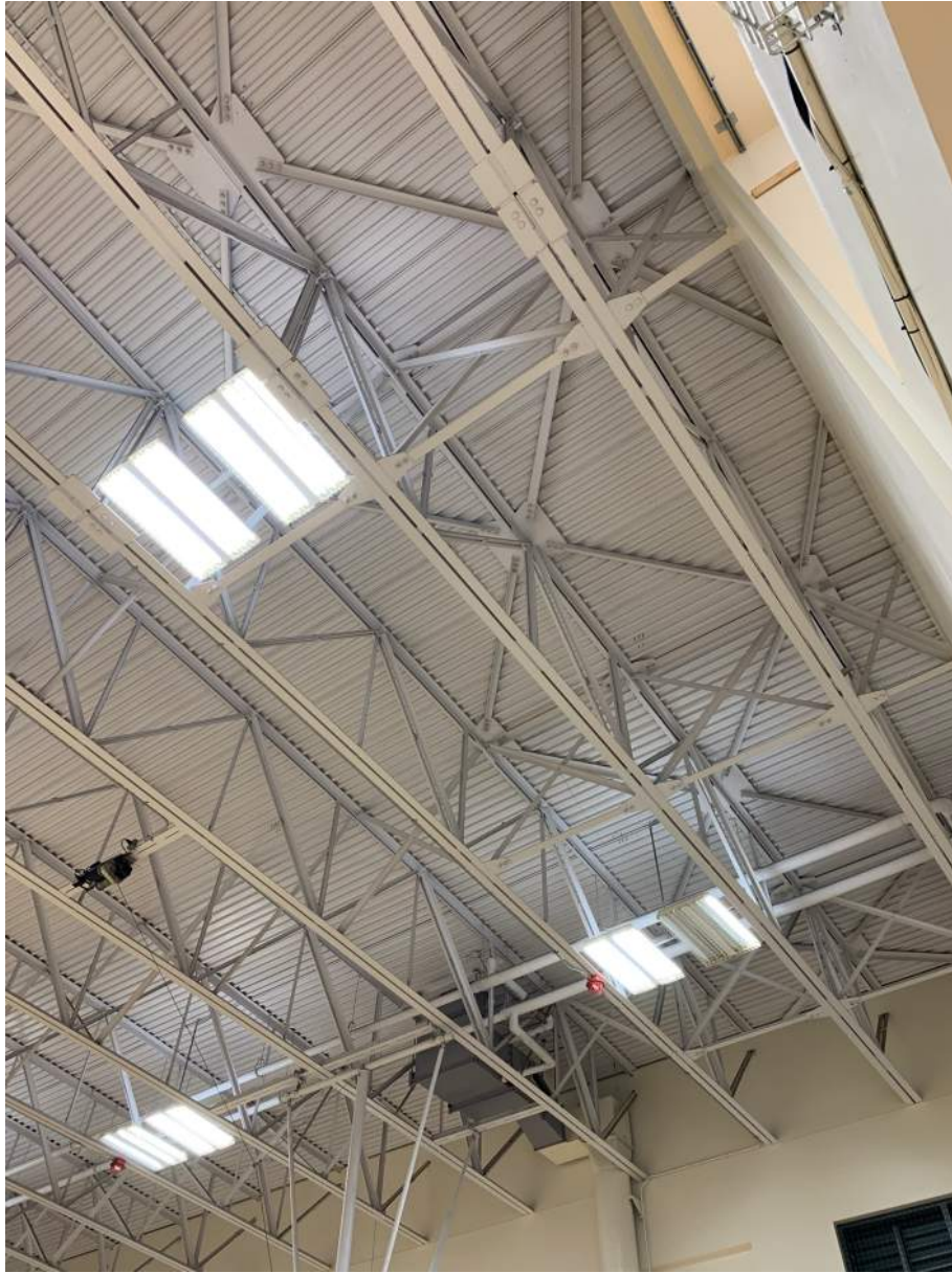
Steel Trusses and Underside of Roof
