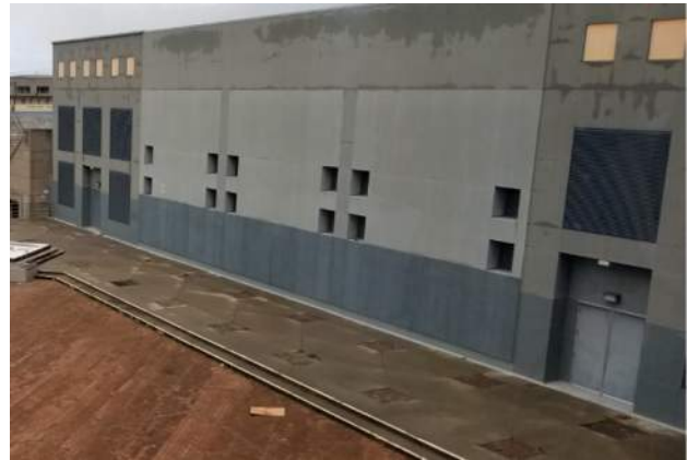
South Elevation Photo
