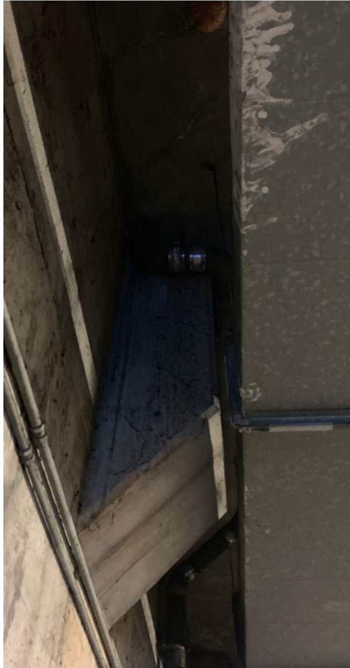
Haunch Supporting Braced Frame Columns
