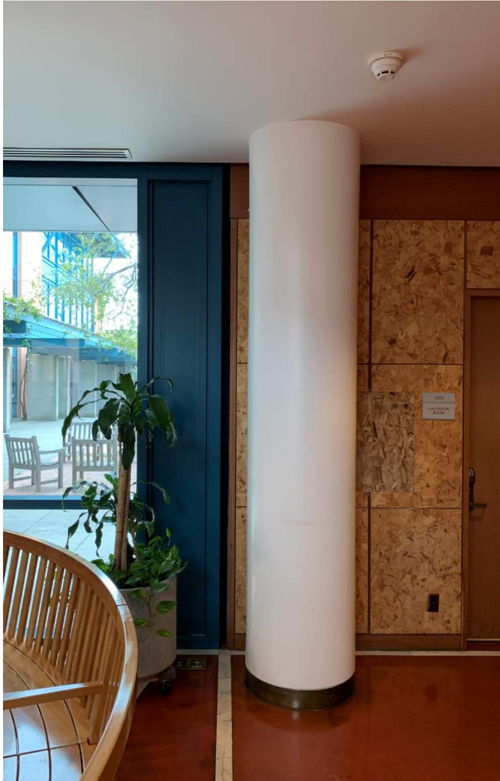
Figure 2 Seismic joint from the interior of the structure
