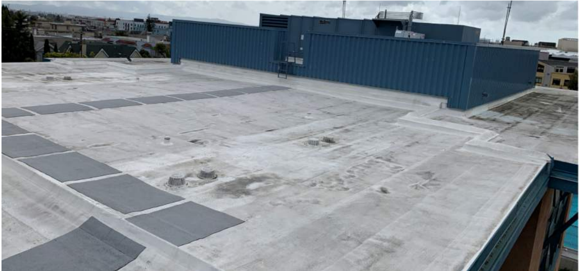
Figure 1 Seismic joint at roof between main structure and west wing
