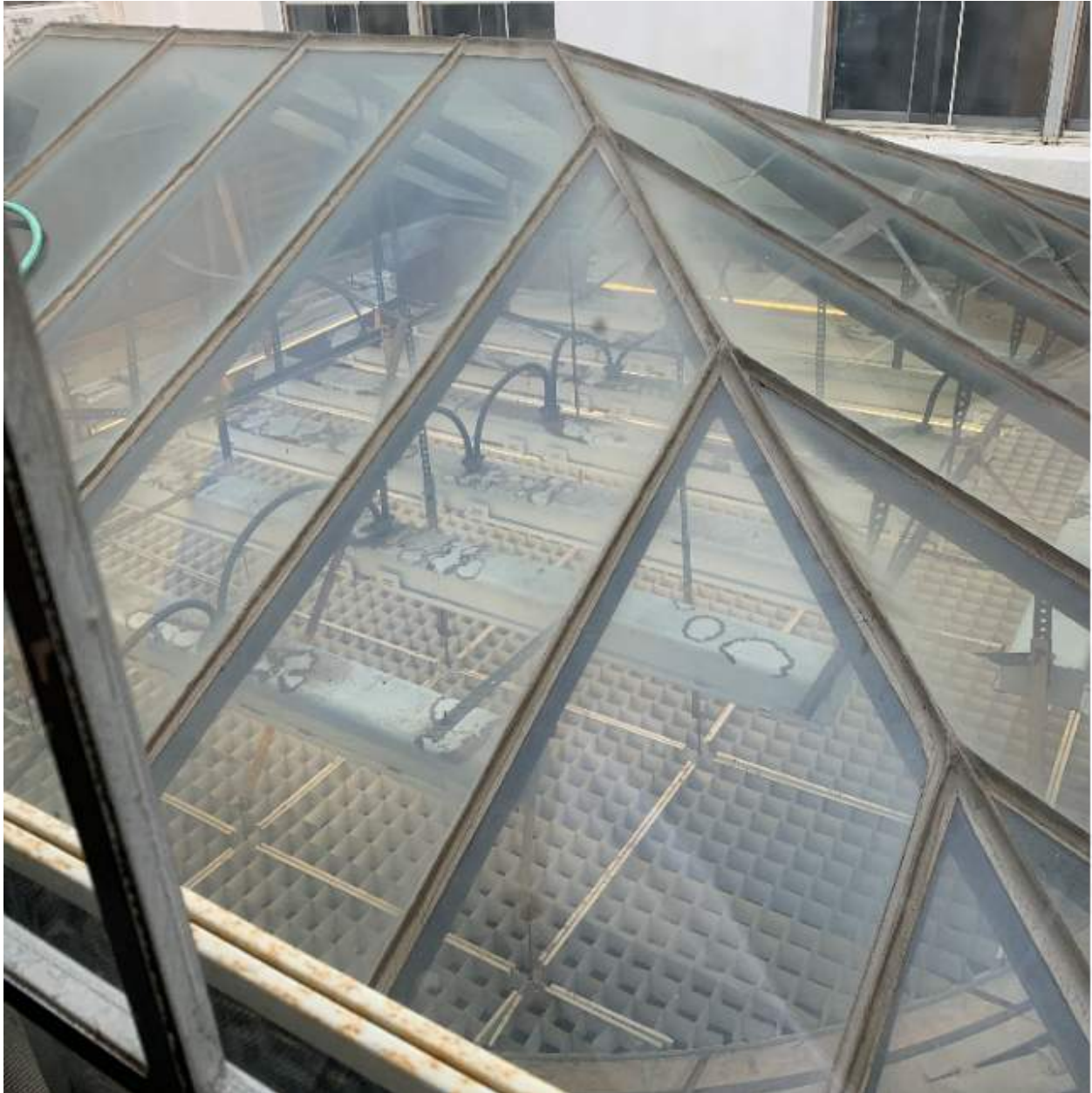
Figure 5 Glass skylight in the North and South Wings
