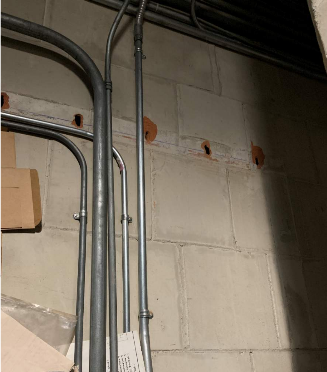
Figure 4 Hollow Clay Tile Used as Partitions in Basement
