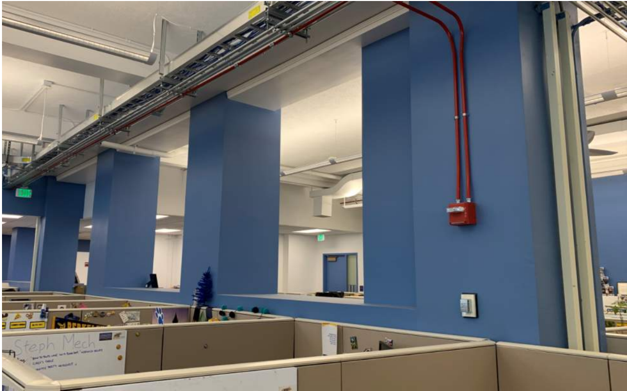
Figure 1 Columns at 1st story supporting discontinuous shear walls above
