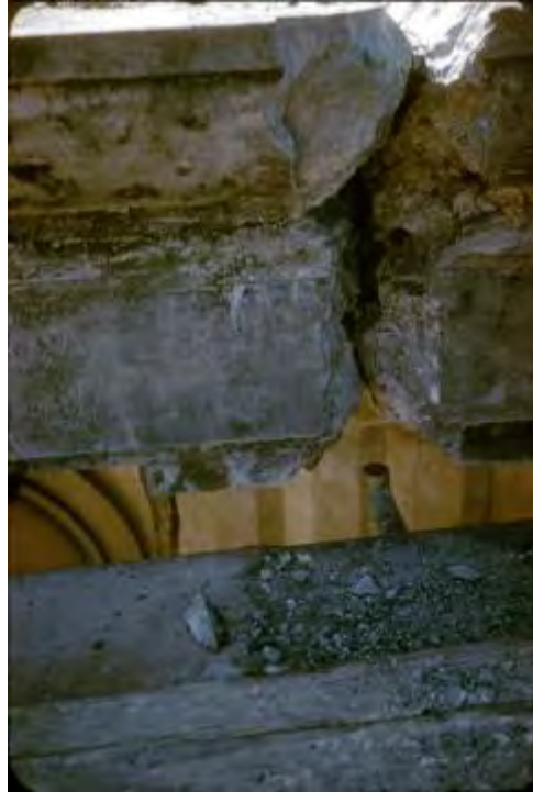
Image 28. This photograph, dated 1954-55, was taken of cornice damage to the stage. It was one of a series of images taken by Water Steilberg of repair work to the theater. Image courtesy of the Environmental Design Archives, University of California, Berkeley.
