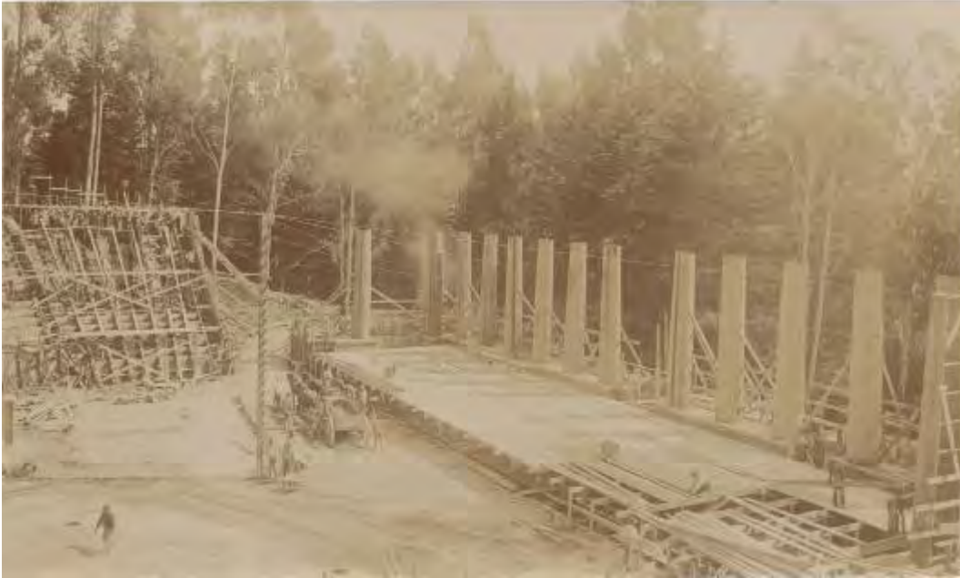
Image 12. May 8, 1903 view of the stage construction, illustrating some tasks in the construction sequence of the stage: the lower stage walls were built first, the column formwork was erected (shown) separate from the stage walls behind, and a temporary wood floor was built in the location of the current stage floor to serve as a working platform for the stage wall construction. Subsequent to the stage construction, the orchestra circle in front of the stage was excavated to its current level. Image courtesy of The Bancroft Library, University of California, Berkeley.
