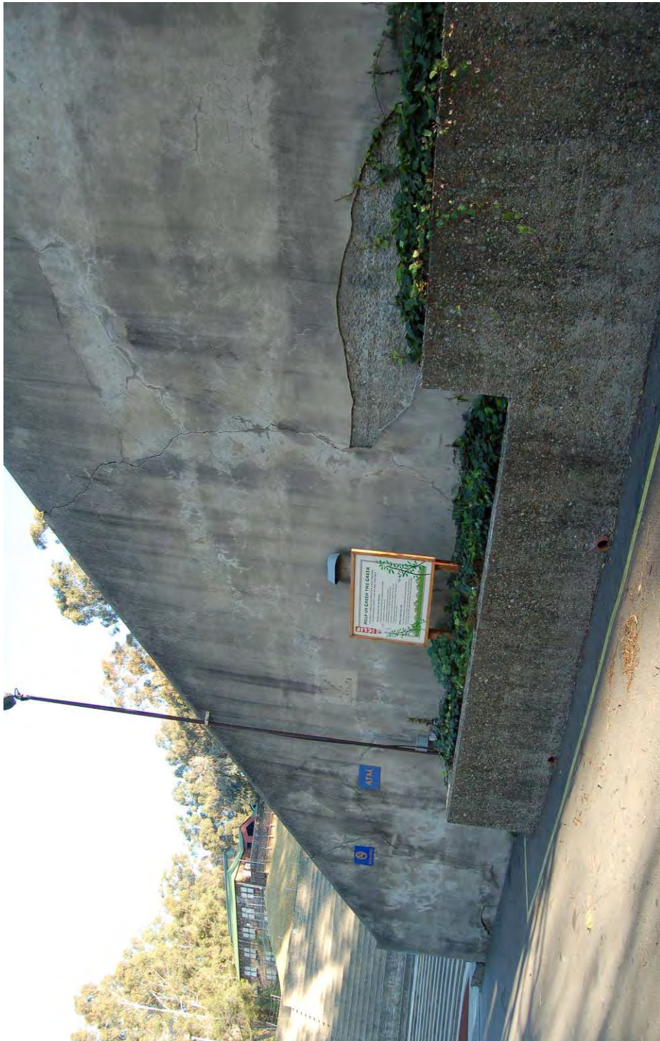
Image 56. South Wall of amphitheater, 2007. Note deterioration in cement coating. Will Dickinson photograph.
