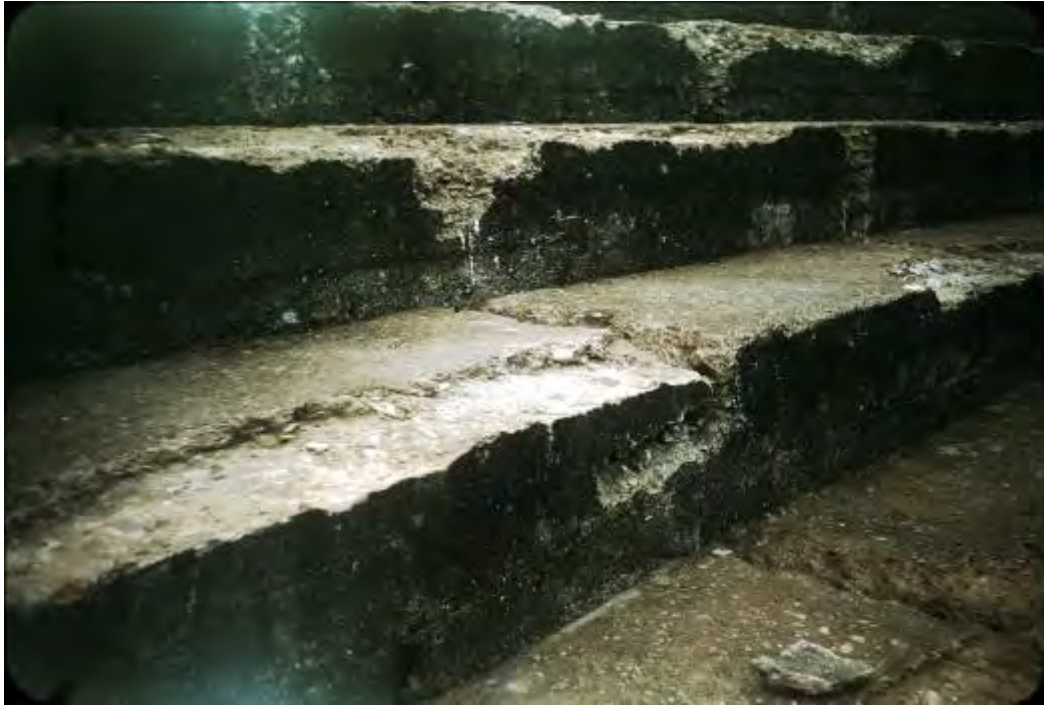
Image 31. This photograph, dated 1954-55, is a close-up view of concrete preparation (the removal of deteriorated concrete) to the amphitheater seating. Image courtesy of the Environmental Design Archives, University of California, Berkeley.
