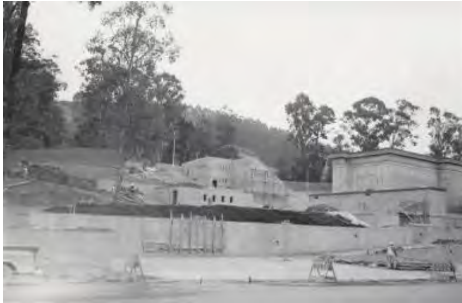
Image 43. View taken in 1957, showing the site during construction. Memorial Plaza is in the foreground, the ticket office is in the middle ground and the ramps and the public toilet room addition to the amphitheater are shown above the ticket office in the background. The scaffolding against the north end wall of the amphitheater suggests the end wall was repaired or coated at this time. The image illustrates the location of repairs to the exterior stage walls, before the application of the cementitious coating, and the infilling of the two blind openings in the return. Image courtesy of The Bancroft Library, University of California, Berkeley.
