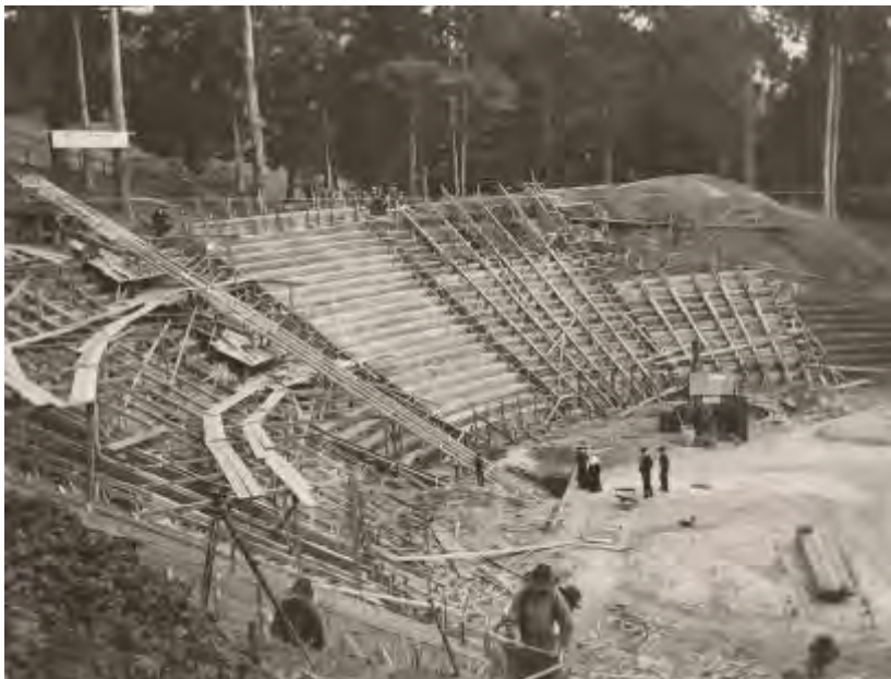
Image 13. View, dating to 1903, of the amphitheater seating under construction, showing the substantial amount of fill used in creating the raked seating and terracing of the earth under the seats. Image courtesy of The Bancroft Library, University of California, Berkeley.
