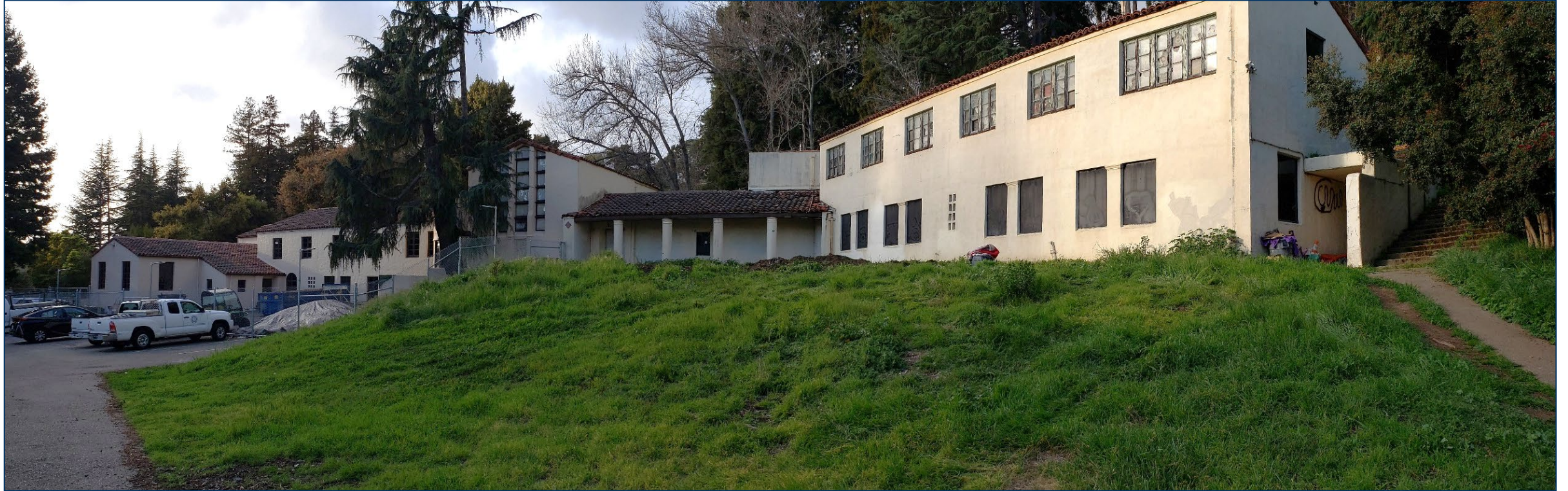
Image 5: Building #21, existing conditions, northwest wing removed (2019)
