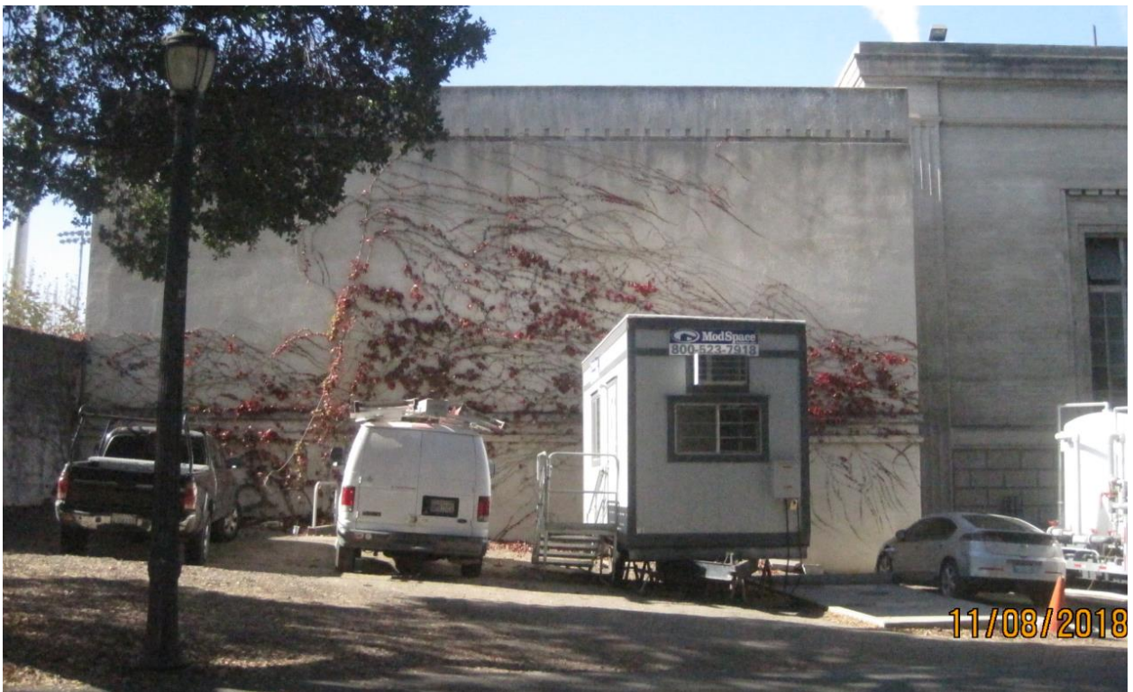
Figure A.2 East Elevation of Cogeneration Plant, specifically. Note lack of openings that is common for the east, south and west faces.
