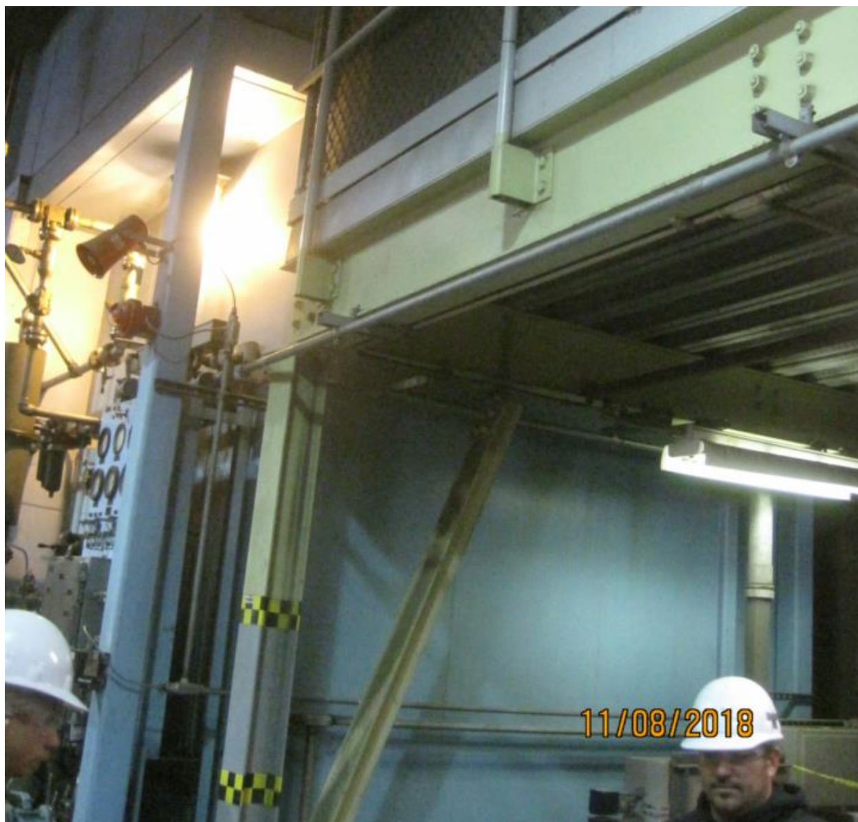
Figure A.4 West Mezzanine (note concentric brace – vertical slotted bolts can just be seen at top of brace)
