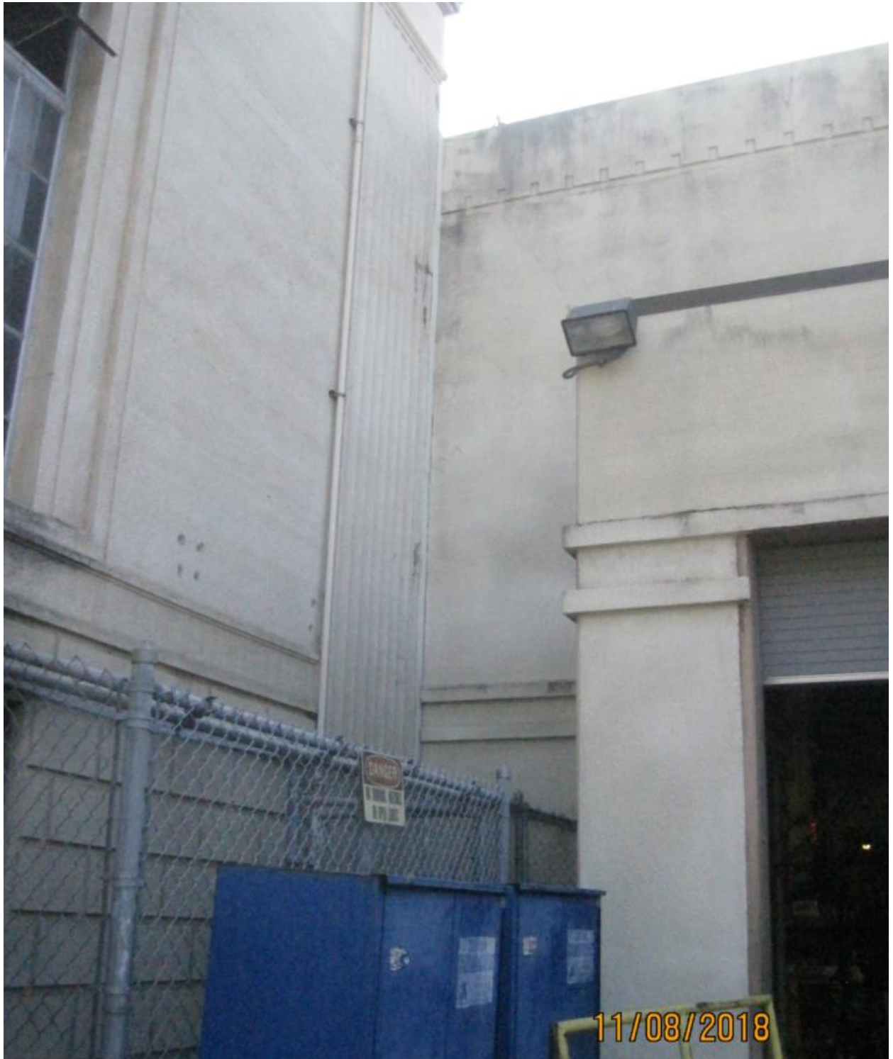
Figure A.3 Intersection of Central Heating Plant (at left) and North face of Cogeneration Plant (at right) (note vertical gray line which covers the 4" seismic separation between the buildings)
