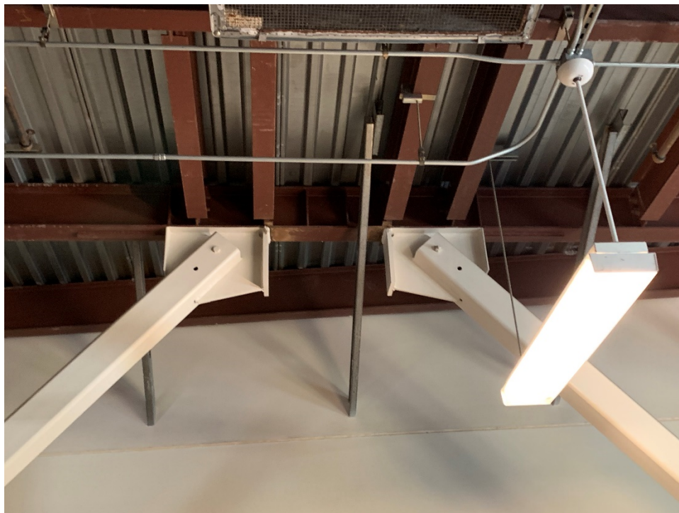
Typical Eccentrically-Braced Frame Top Connection
